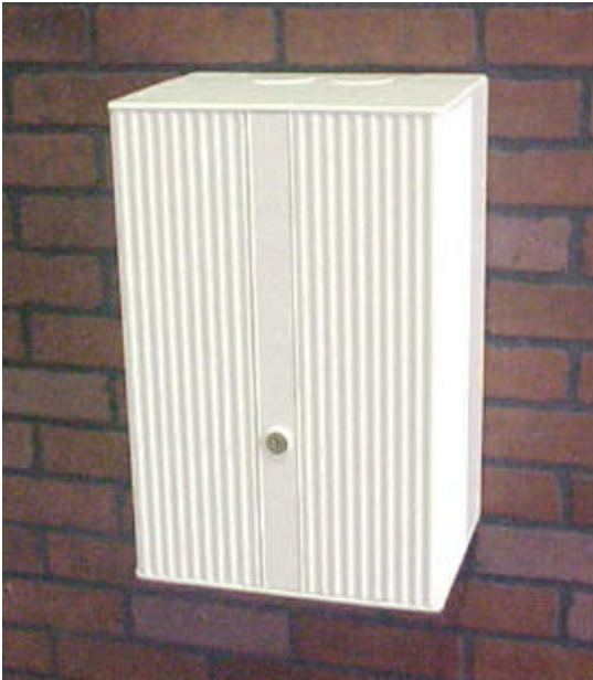
Standard BOSS mounted on Apartment Complex
